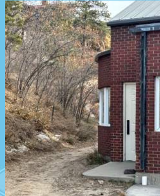
Narrow space between MS and steep rocky incline (6-10 feet) is inadequate to install Drainage Solution.
