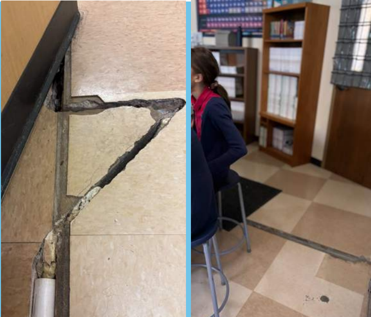
2" wide x 6" deep floor crack in Science Room filled with grout continues to grow in 2025
