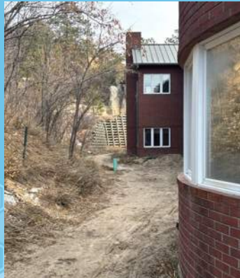
Narrow space between MS and steep rocky incline (6-10 feet) is inadequate to install Drainage Solution.
