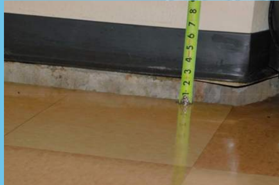
Floor slab settlement over 2 inches
