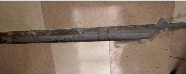
2" wide x 6" deep floor crack in Science Room filled with grout continues to grow in 2025
