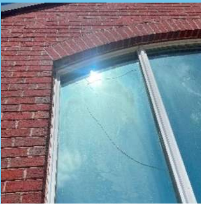
Windows crack due to foundation movement
