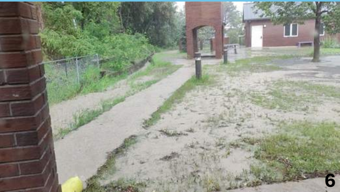
6-inch Area Drain is inadequate to convey flows from +3.5 acres above; Images from 2023 storm video – link in grant text
