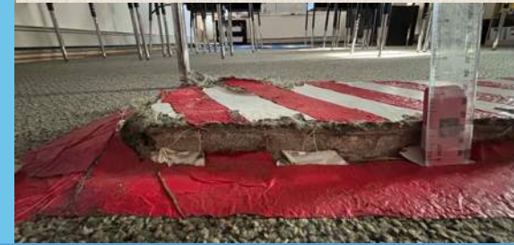
Grade beam protrudes 1" above settled slab, tripping hazard, ADA violation
