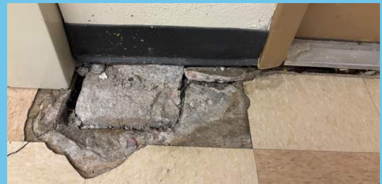
Floor slab distress at Middle School
