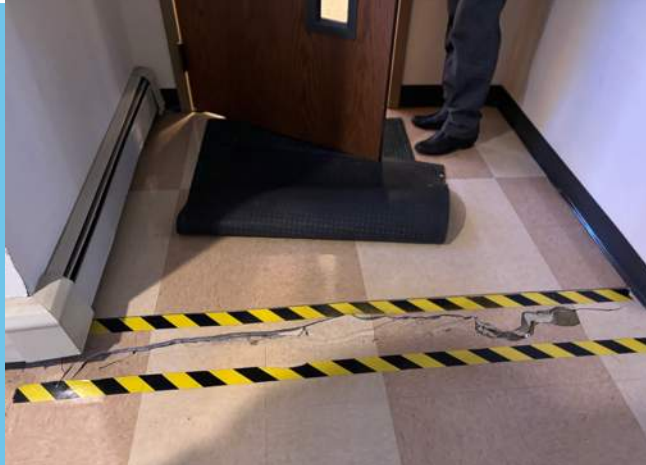
Crack in Middle School hallway continues to fracture slab and increase in size and depth
