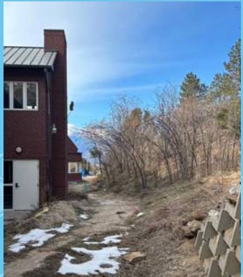
Narrow space between MS and steep rocky incline (6-10 feet) is inadequate to install Drainage Solution.
