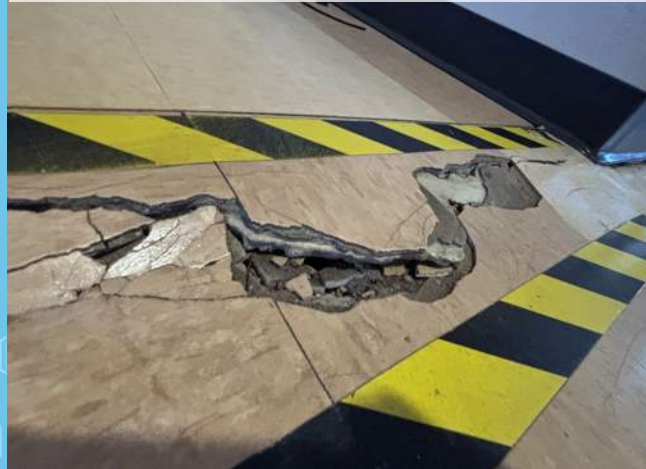
Crack in Middle School hallway continues to fracture slab and increase in size and depth
