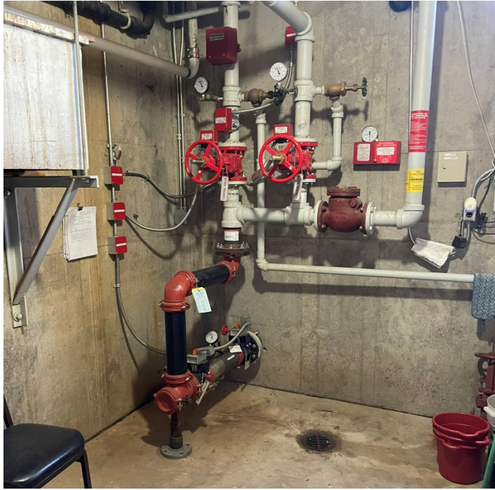
Image 10: Existing Fire Riser Room in the Elementary School basement
