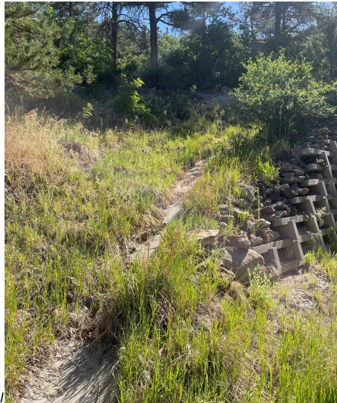
Image 4: Existing Retaining wall concrete rundown
