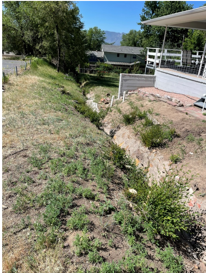
Image 12: Existing Ditch where flooding causing erosion to adjacent residence
