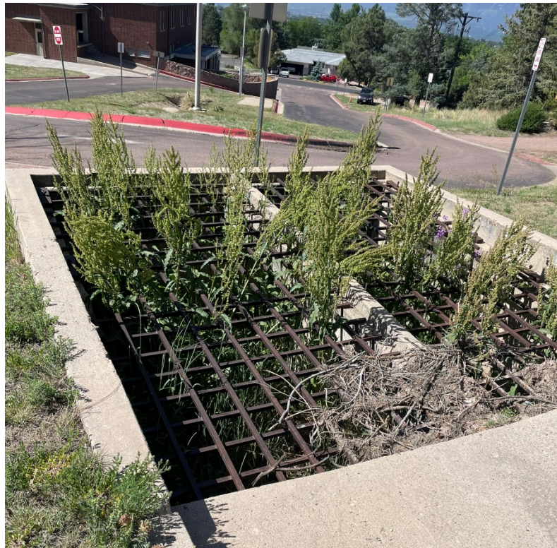
Image 10: Existing stormwater inlet
