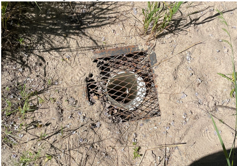
Image 6: Existing 6" area drain behind MS rear at base of concrete pan
