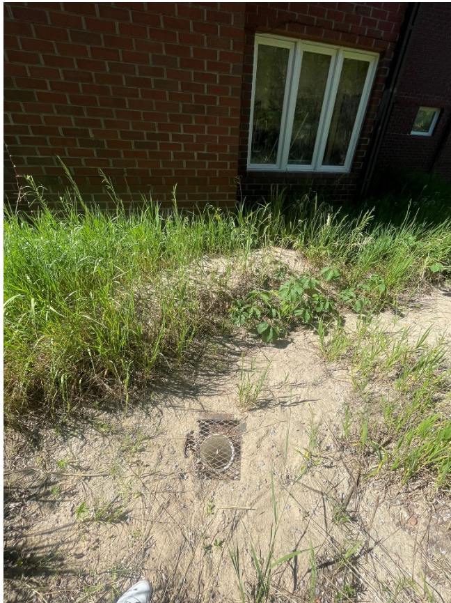
Image 8: Existing manmade berming adjacent to MS at base of mountain and area drain
