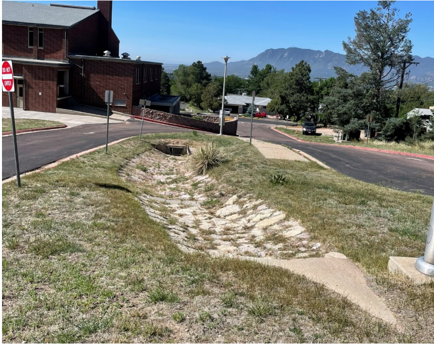
Image 11: Existing Storm ditch downstream of inlet
