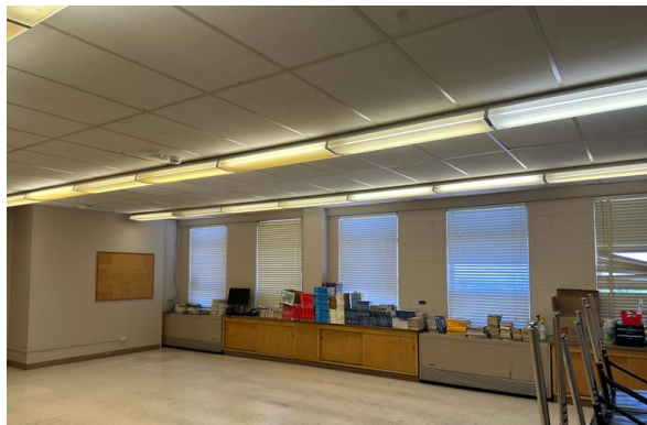
Original classroom luminaires T8 lamps
