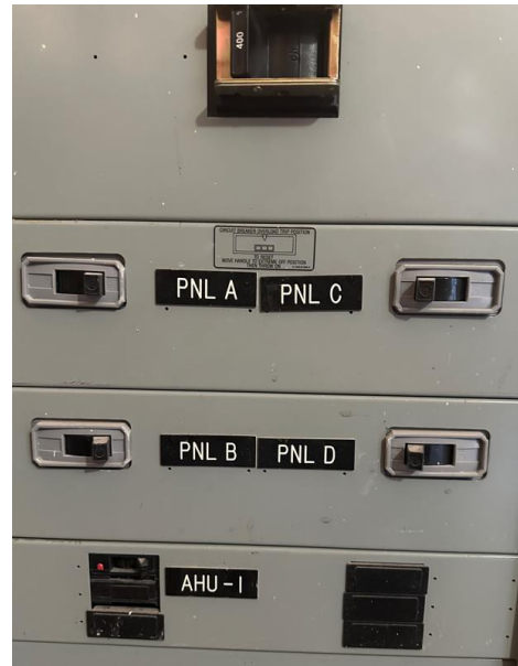
Main Distribution Panel in Mechanical/Electrical Room
