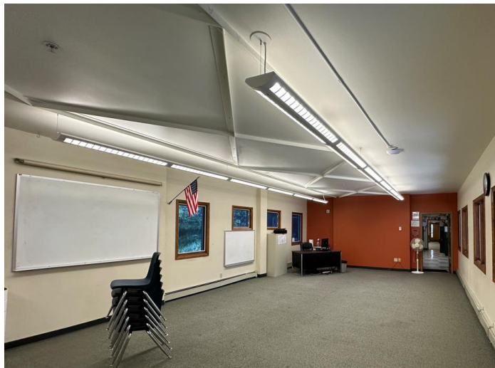
Cable hung direct/indirect classroom lighting
