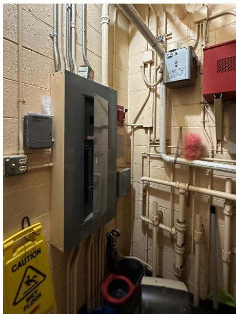
Main electrical panel in janitor's closet
