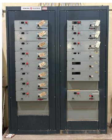
Switchboard with fused disconnects for mechanical systems
