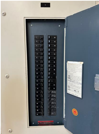
Corridor recessed branch panelboard
