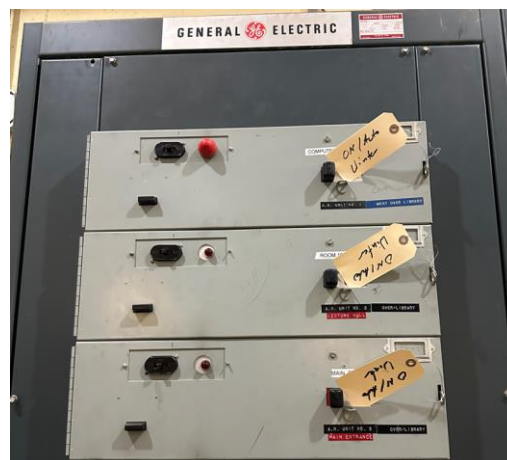
Switchboard with fused disconnects for mechanical systems
