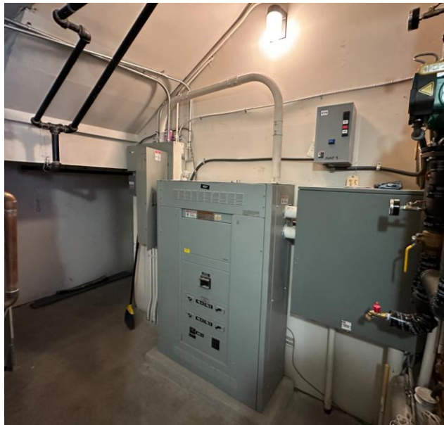
Main Distribution Panel in Mechanical/Electrical Room
