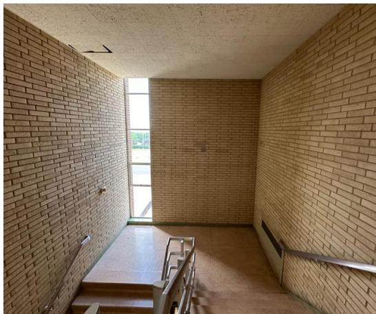
Stairwell with missing wall luminaire
