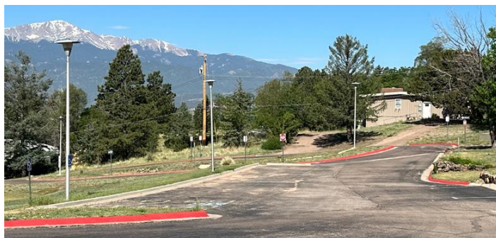
Not full cut-off pole mounted luminaires at parking lot
