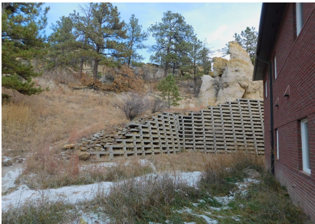
7. Northeast corner of the building. Crib retaining wall and poor drainage conditions.
