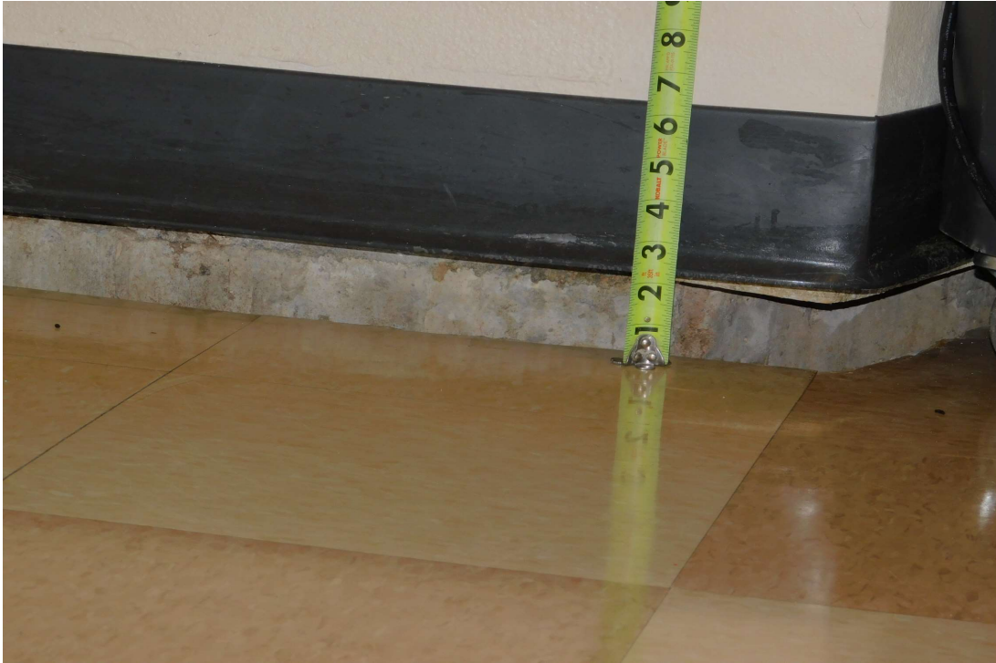
15. Slab settlement at northwest corner of the science room.
