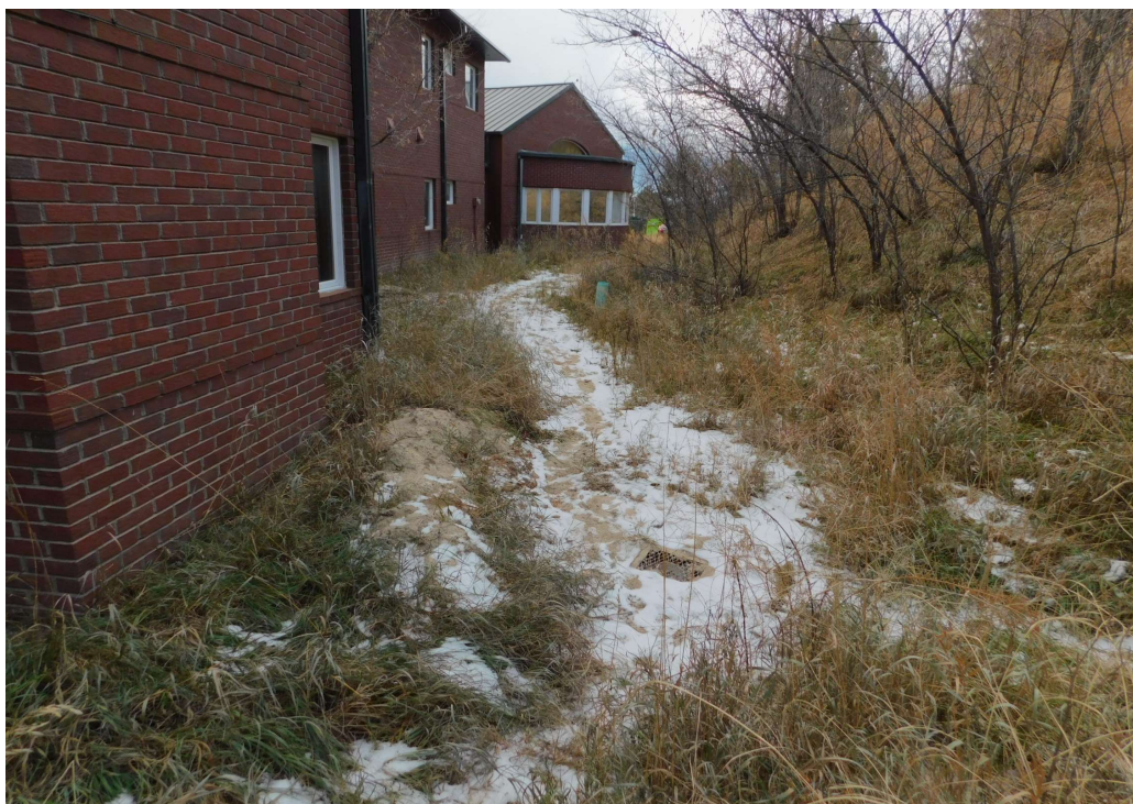
5. North side of the building viewed from outside of the north wing foyer. Existing poor drainage conditions throughout the area.
