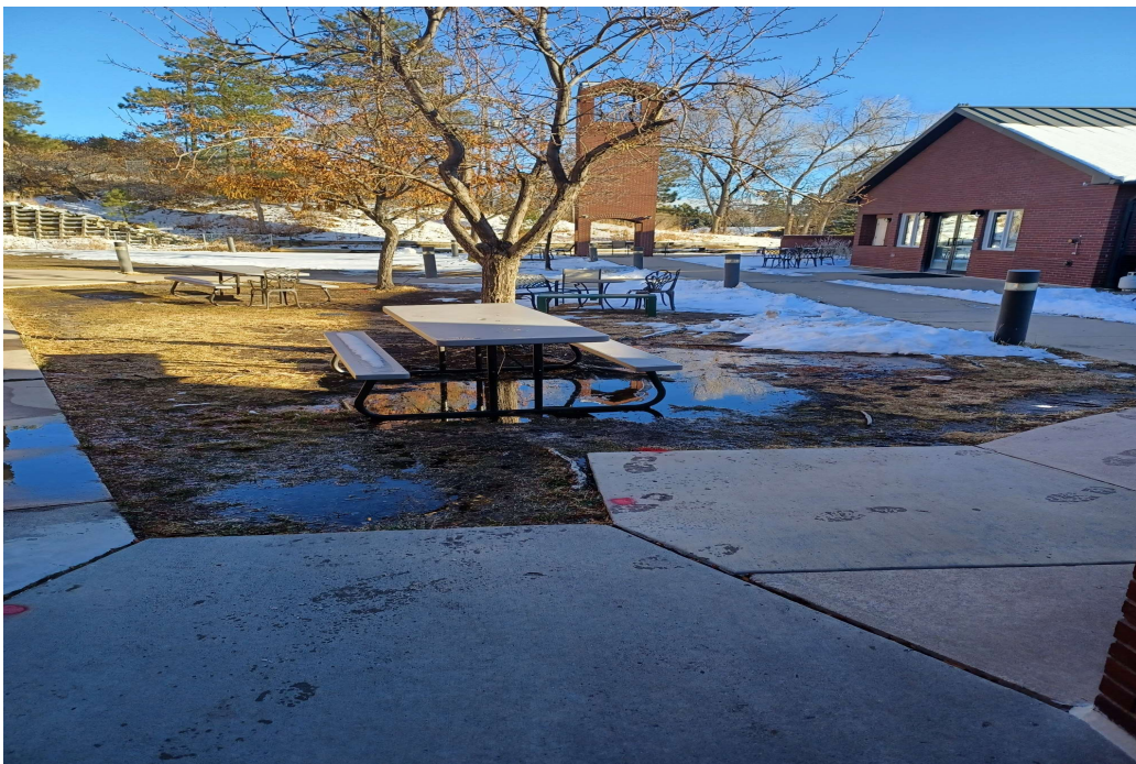
10. Poor drainage within the patio/courtyard.
