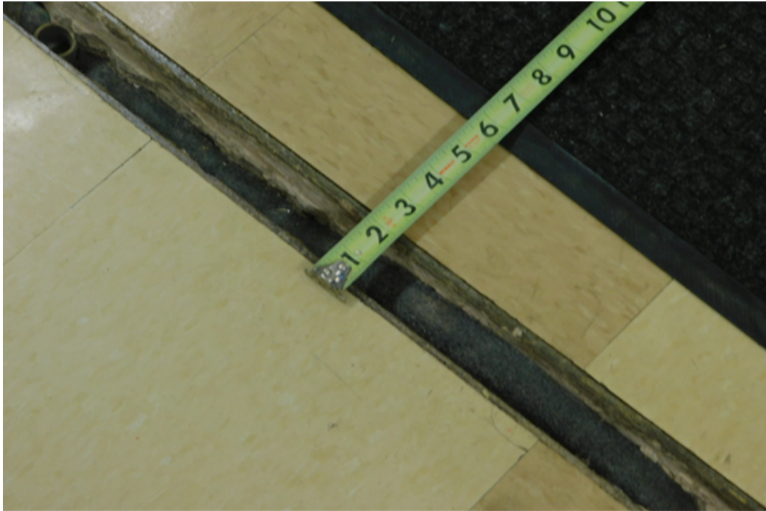
13. Floor slab separation in science room.
