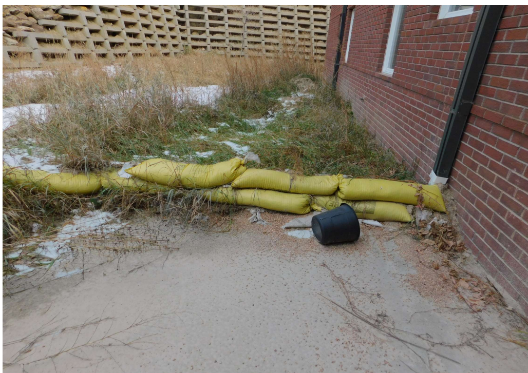
8. Poor drainage patterns along north side of the school.
