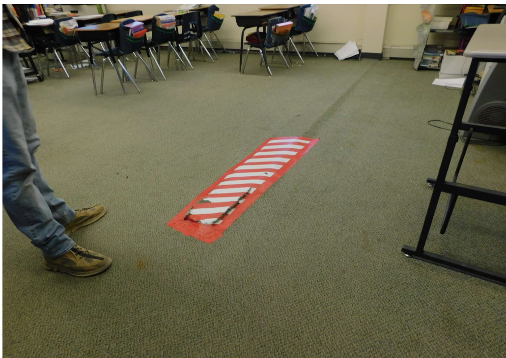
11. Vertical displacement of floor slab at grade beam in classroom 308.
