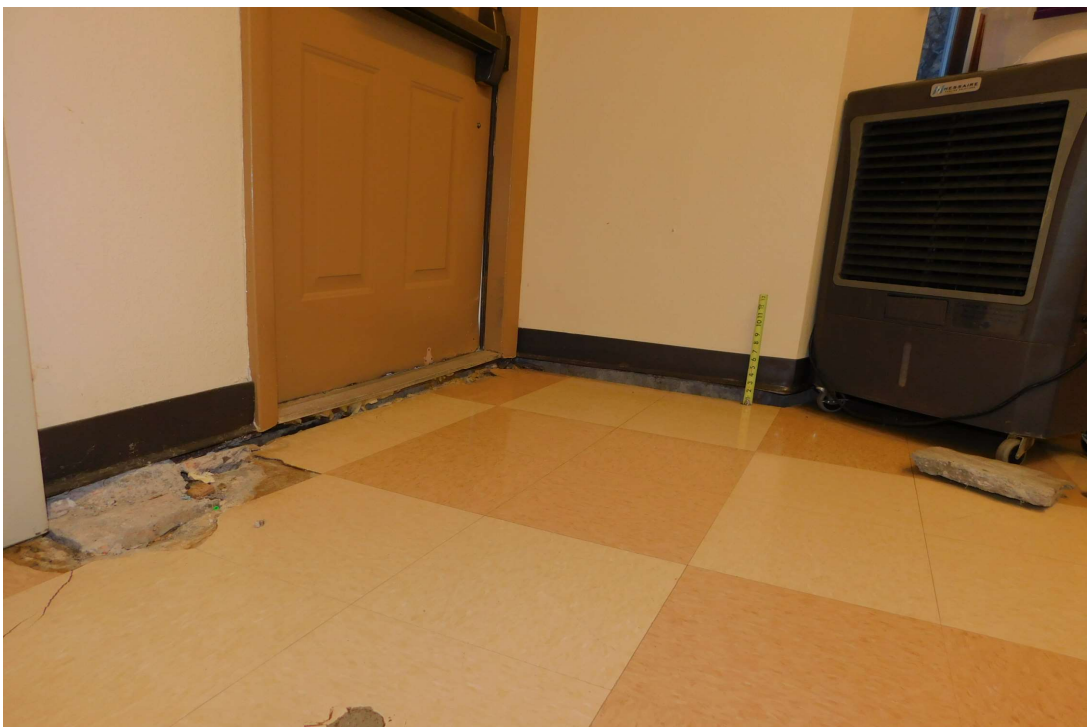
14. Slab damage at slab edge located at the northwest door of the science room.
