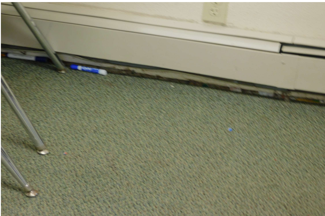
16. Slab settlement at slab edge.
