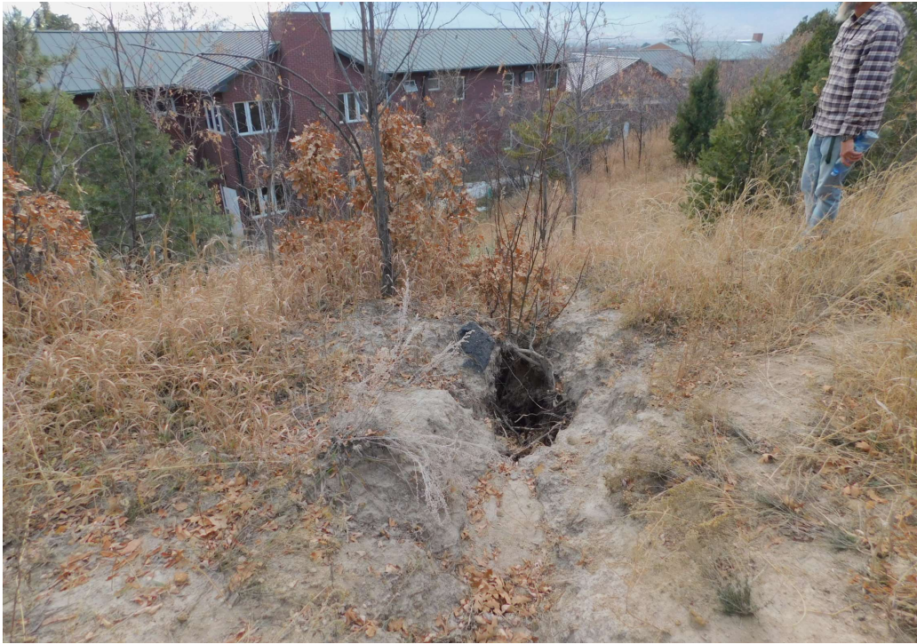
9. Stormwater pond on slope of Palmer Park. Erosion channel forming from uncontrolled stormwater runoff from the slope and out of pond toward school building.
