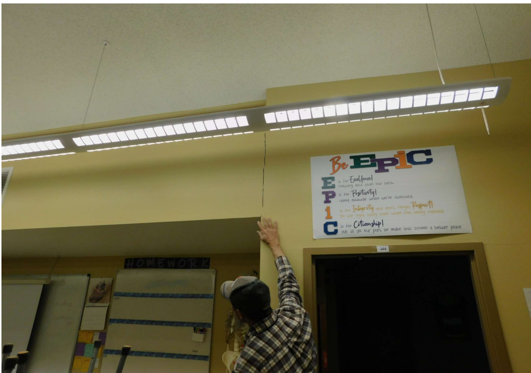
18. Drywall joint crack at door to science room.
