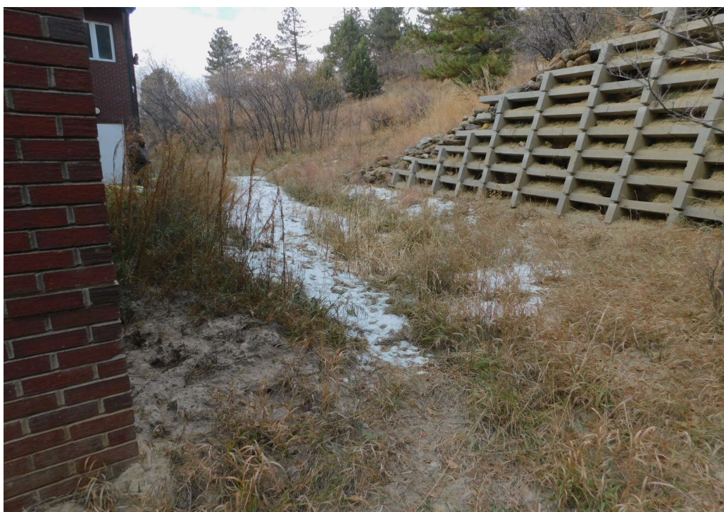
4. View of the north side of the building from near the northeast corner. Concrete crib retaining wall present on the right. Poor drainage conditions throughout.
